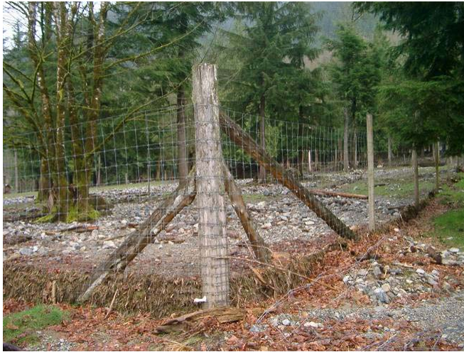
Debris flood: Peak discharge bulking factor: 1 to 2 x peak discharge of a water flood
