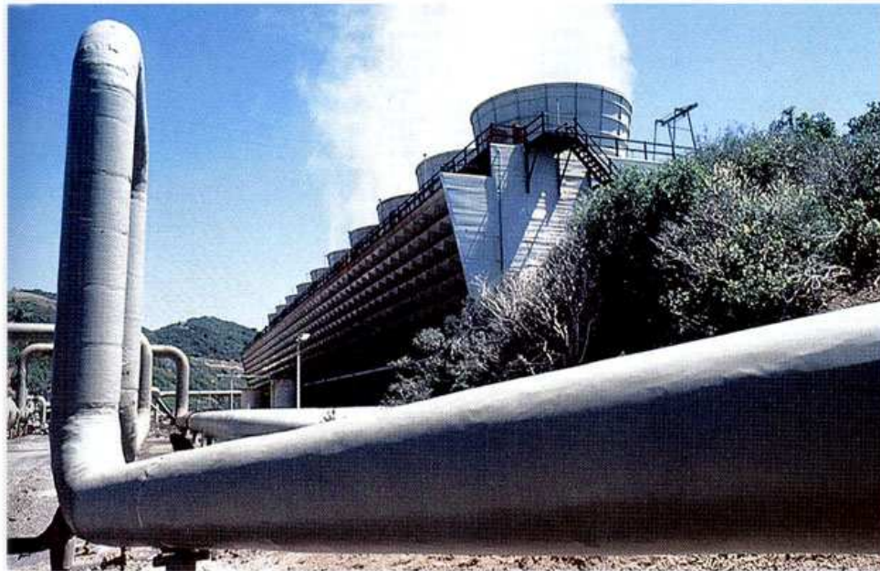
◀ FIGURE 15-23 Geothermal energy. One of the 11 geothermal units operated by the Pacific Gas & Electric Company at The Geysers in Sonoma and Lake counties, California. California geothermal energy produces 1,600 MW of power, roughly 7% of California's energy needs.
